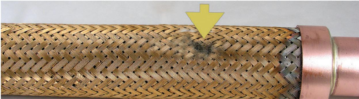
The faint dark area on this vibration eliminator is evidence of oil-refrigerant seepage.
